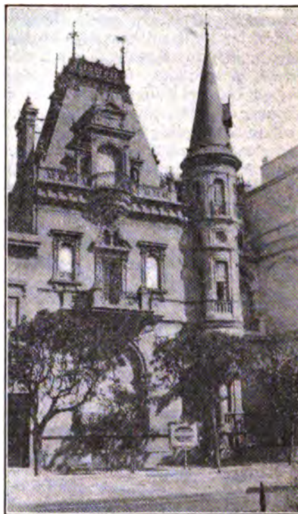
This façade won the prize for the best building erected in 1908
